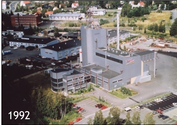
80 ton per day Gasification Pilot Plant in Tampere, Finland using biomass & coal
