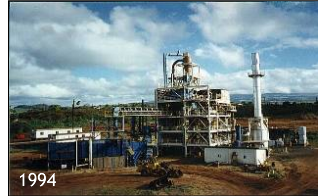
100 ton per day Bioenergy Demo Plant in Maui, Hawaii using bagasse
